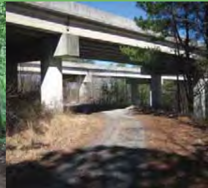
Fig. 34 - Existing Access for Trail under I-575 Courtesy of: Ecos
