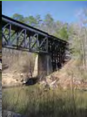
Fig. 36 - Trestle Bridge Courtesy of: Ecos
