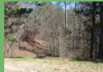
Fig. 48 - Sewer easement at Woodstock Middle and High School Courtesy of: Ecos
