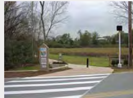
Fig. 58 - Typical Trail/Road Intersection Courtesy of: PATH Foundation
